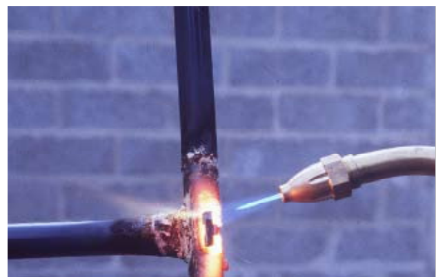
Figure 4.4 Construction – Use of silent blowtorch (© Yves Cousson – Courtesy of INRS – France)
